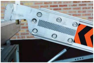
Stress points are taken care of with a longer arm and multiple fasteners.
